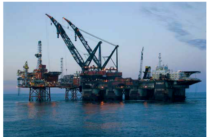
Crane barges use DP to good advantage. Here Thialf is at work in the Captain field
