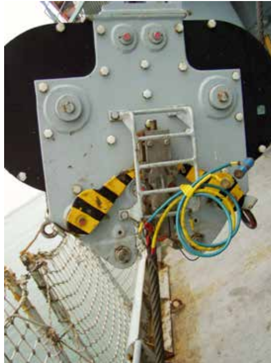
Fig 7F-7. Cables and toggles secured to steel guard
