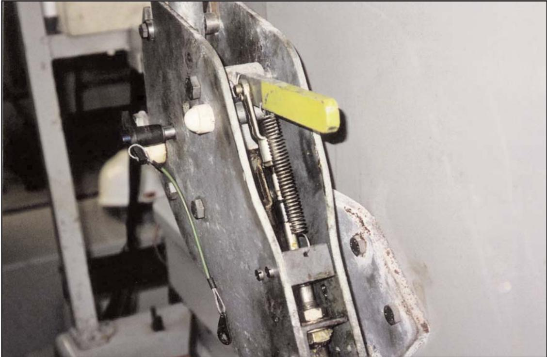
Interlock lever with protective cover removed
