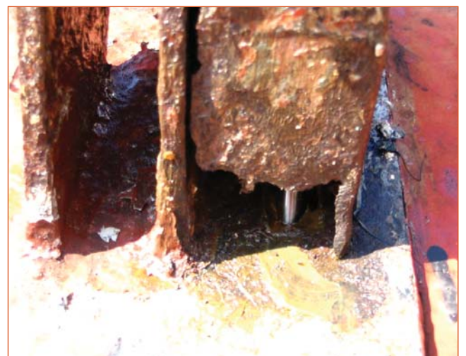
CORROSION AND WASTAGE
