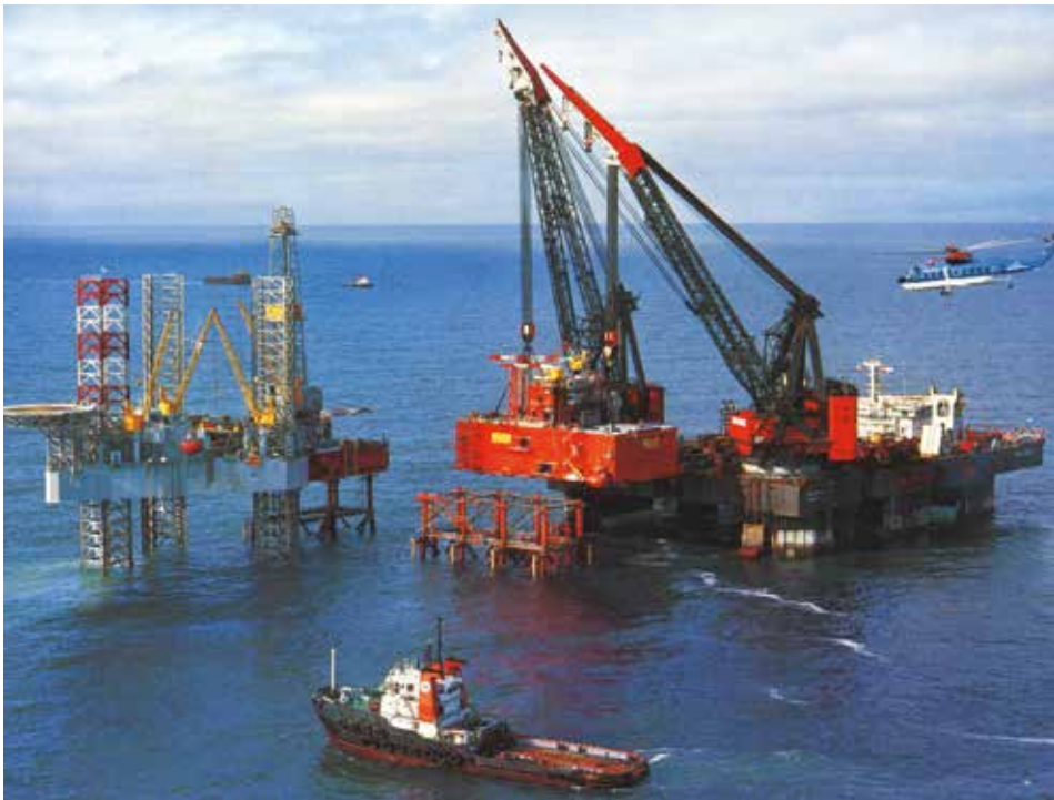
Offshore construction vessel Balder positioned for a topside installation
