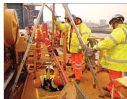
▲ An example of a difficult access. It is not possible to wear any type of BA set to enter this compartment
